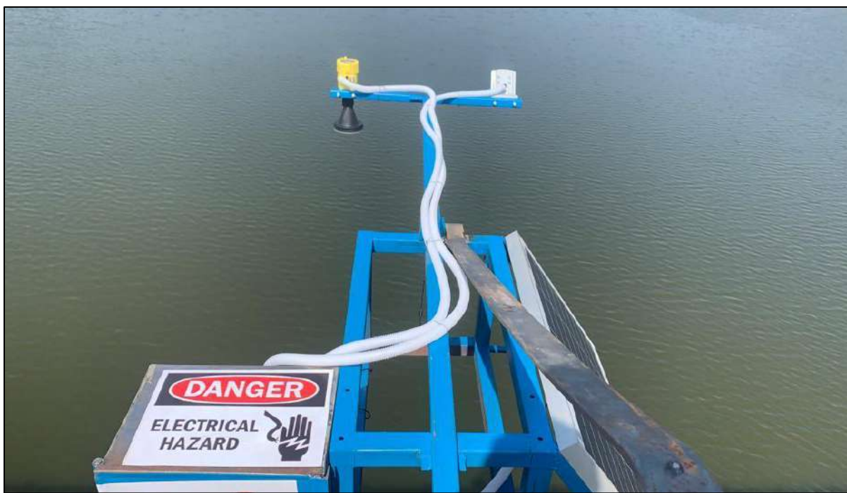
4. Mannur Bridge Latitude: 17.299832 Longitude: 76.084808
