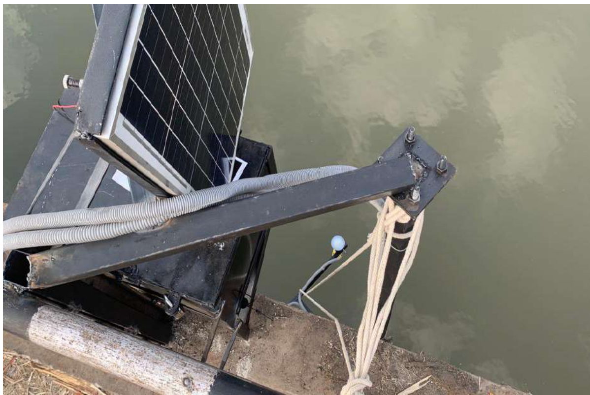
8. Thinthani Bridge Latitude: 16.368032 Longitude: 76.657025
