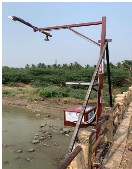
9. Cholechagudda Bridge Latitude: 15.875892 Longitude: 75.721887
